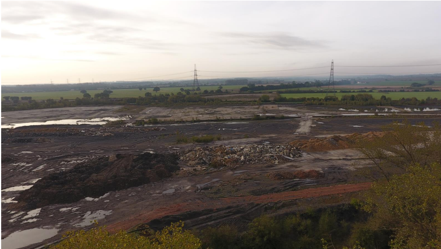
Figure 8: Drone view to the southern part of the site with railway track which runs through the southern part of the site
